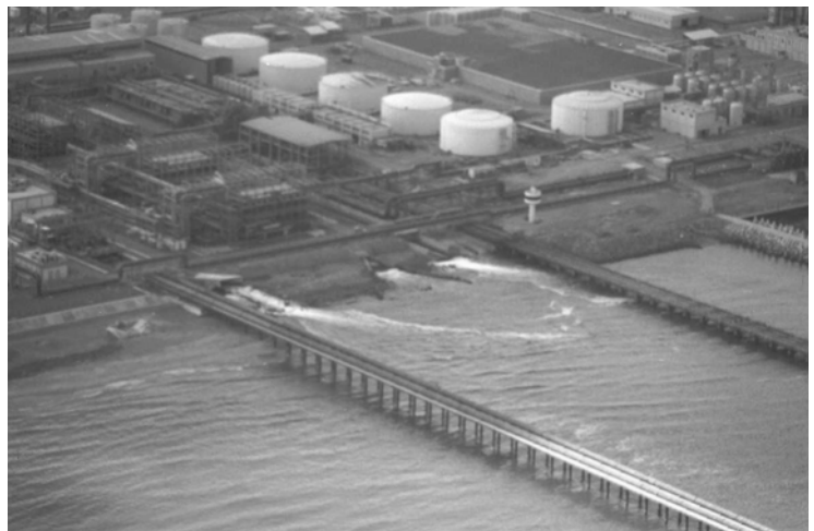
Fig. 1: Al Ghubrah desalination plant (largest in Oman, production capacity 191,000 m 3 /d): Brine waste discharge through an open channel at the beach into the Gulf of Oman (photo: H.H. Al-Barwani)
